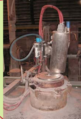
Inspection window and housing for the thermal imaging device
