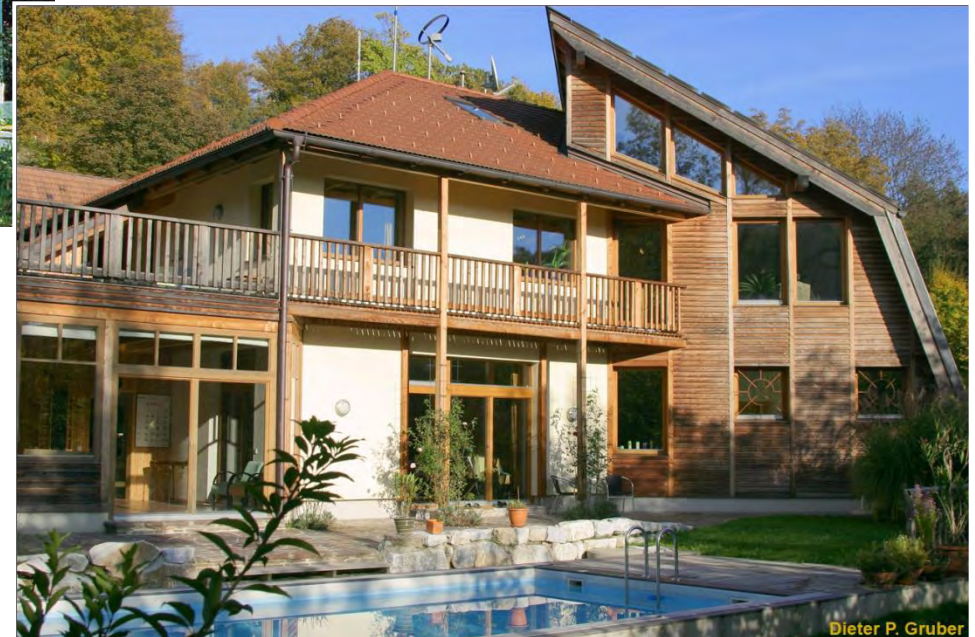
Ultra-low energy solar country house (Graz, A; 1998)
