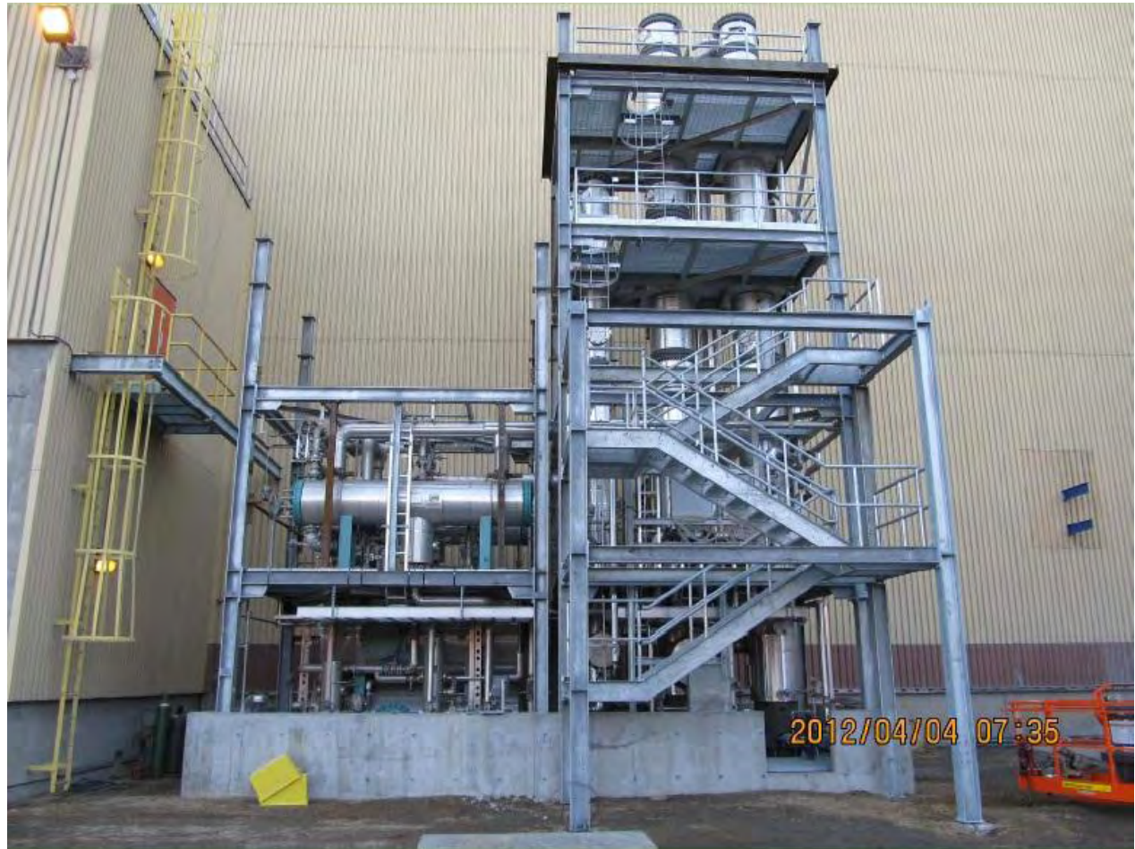
A pulp, off-gas, electricity & heat biorefinery for the production of kraft pulp, biomethanol, electricity and heat from wood chips [Alpac Forest Products Inc., Canada]
