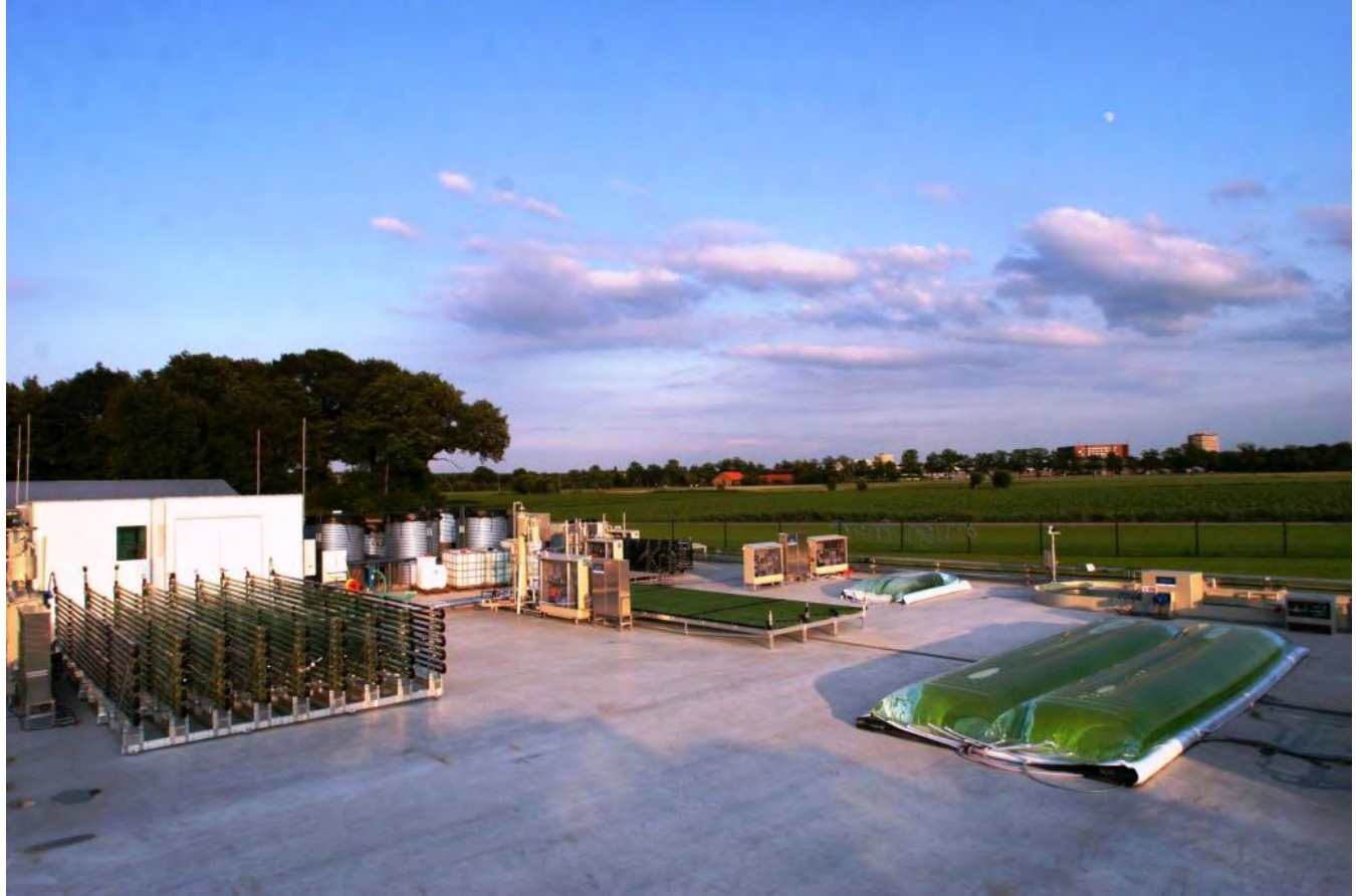
An oil production and refinery pilot-plant for Omega-3, fuels, chemicals from microalgae [Wageningen UR, the Netherlands]
